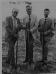
Digging in at the June 8, 1968 groundbreaking for the WBCTC are (from left) Jefferson Davis Campus Vice-President Glen Cagle, MGCC President J. J. Hadden Jr., and WBCTC Administrative Dean Sam Kinch.
