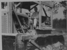
At the groundbreaking ceremony at Jackson County Campus MGCC President J. J. Hadden gets JC off to a meeting start with a bulldozer.
